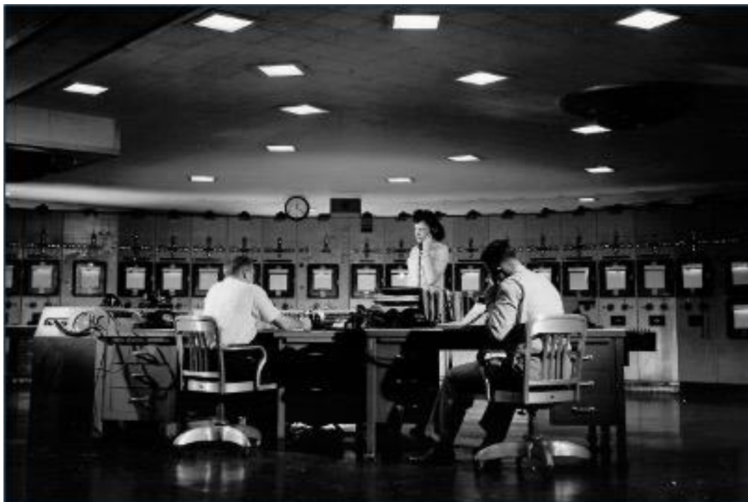
K-25 Gaseous Diffusion Plant, Clinton Engineer Works, Oak Ridge TN The Control Room was the most advanced, most fully instrumented plant of its time. (Public domain Courtesy of Barbara Scollin)
